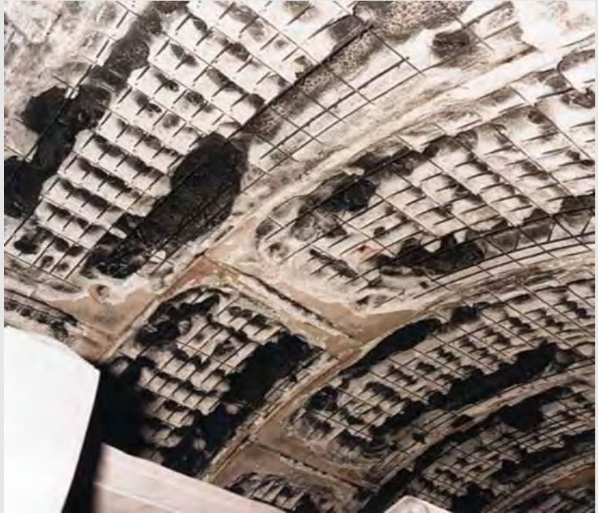
Fire Spalling
